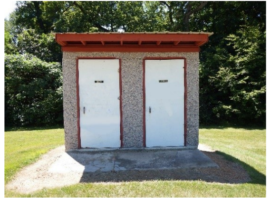
Vault-style restroom facility at Buffalo Creek County Park.
