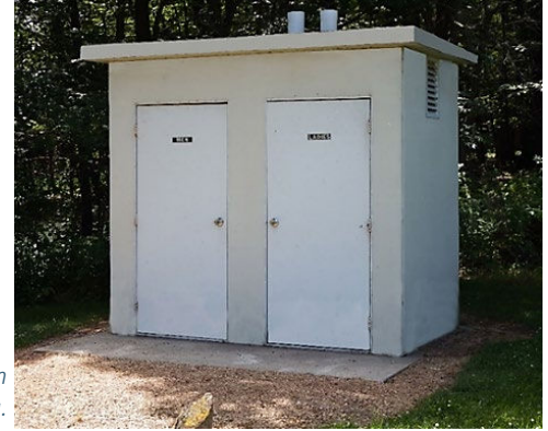
Stahl's Lake County Park restroom facility near the picnic area.
