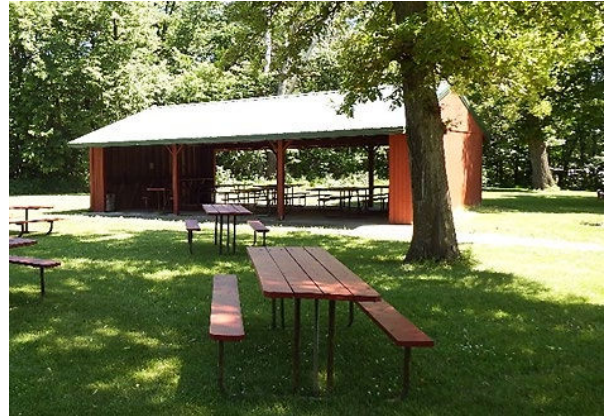
Northern picnic shelter facility at Piepenburg Regional Park.
