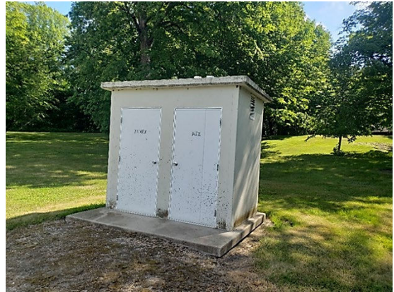
William May County Park restroom facility.
