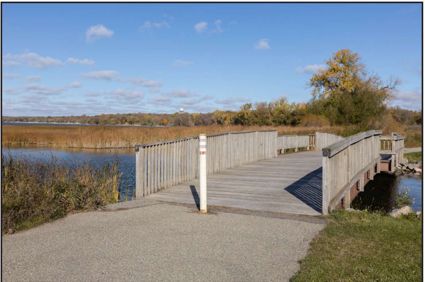
Pedestrian Bridge at Green Lake Outlet/Middle Branch of Crow River
