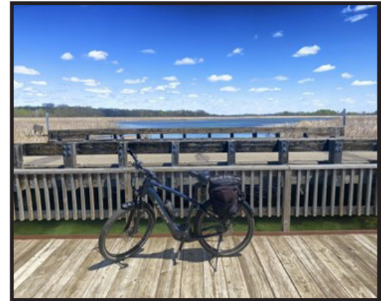
A dedicated bicycle and pedestrian bridge is provided where Green Lake empties into the Crow River. 20 (Above)
