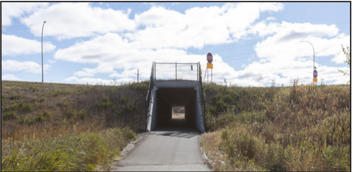
A pedestrian underpass allows trail users to cross U.S. Hwy. 71 and Kandiyohi County Rd. 40 without traffic
