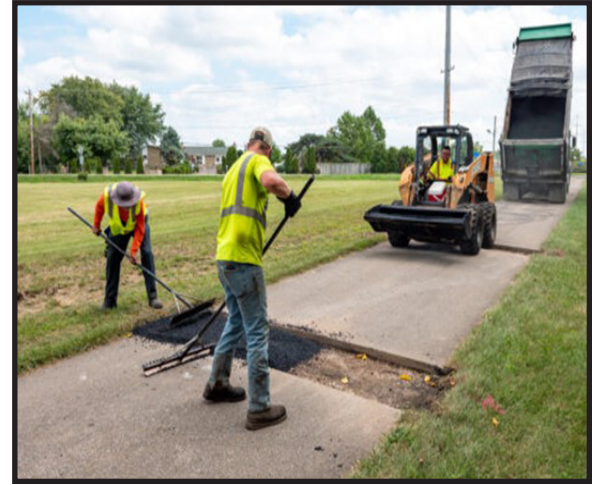
A construction crew repairs a section of paved trail.
