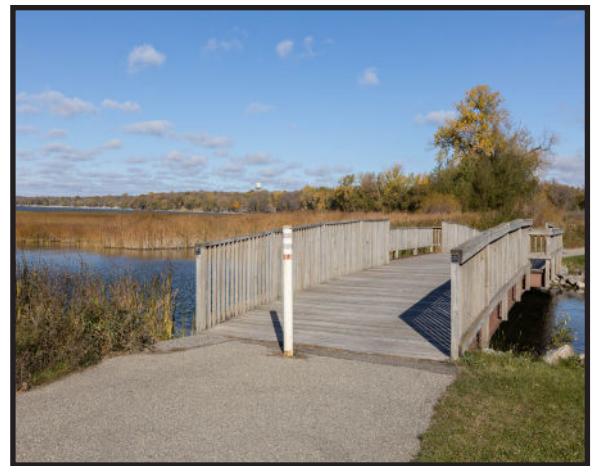
This Bridge, which Crosses the Glacial Lakes State Trail, Provides a Point of Interest between Spicer and New London, MN
